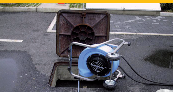
Ventilation positive and negative
